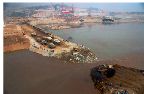
Fig. 7. River closure of the Three Gorges Project.
